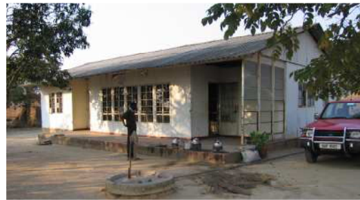
The New RENATO centre
